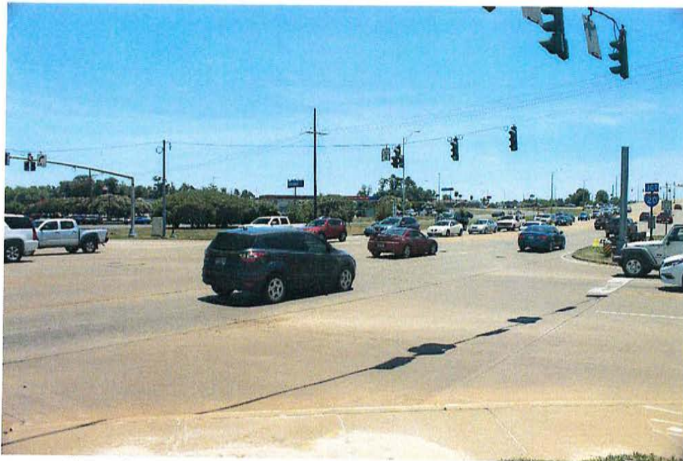
Figure 11: Intersection of Thomas Rd. and Glenwood St. in West Monroe
