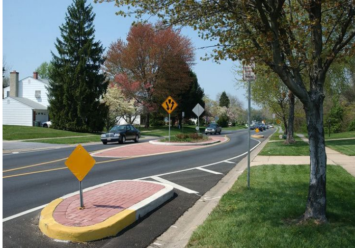
Source: National Association of City Transportation Officials Example of traffic calming measures
